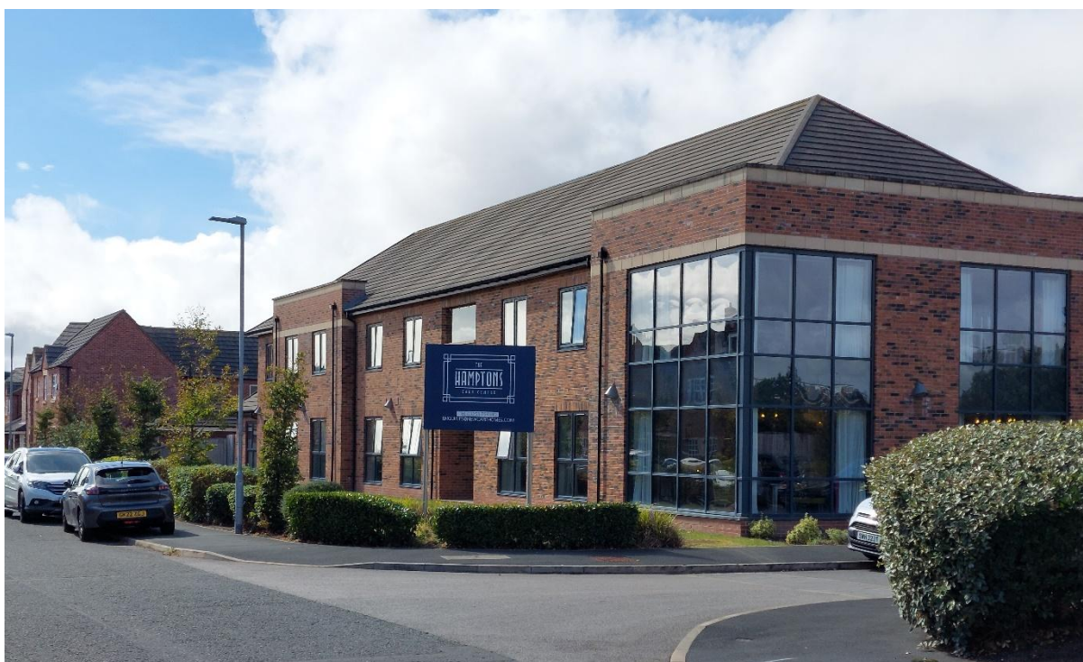
New care home in St Annes constructed as part of a larger housing development
