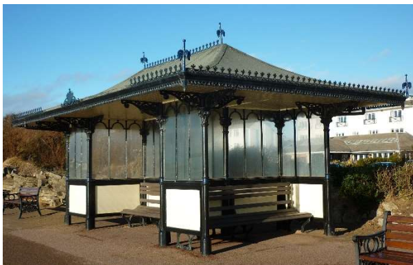
One of the two cast iron shelters by McDowall, Steven & Co. Ltd of the Milton Foundry, Glasgow erected C1908.
