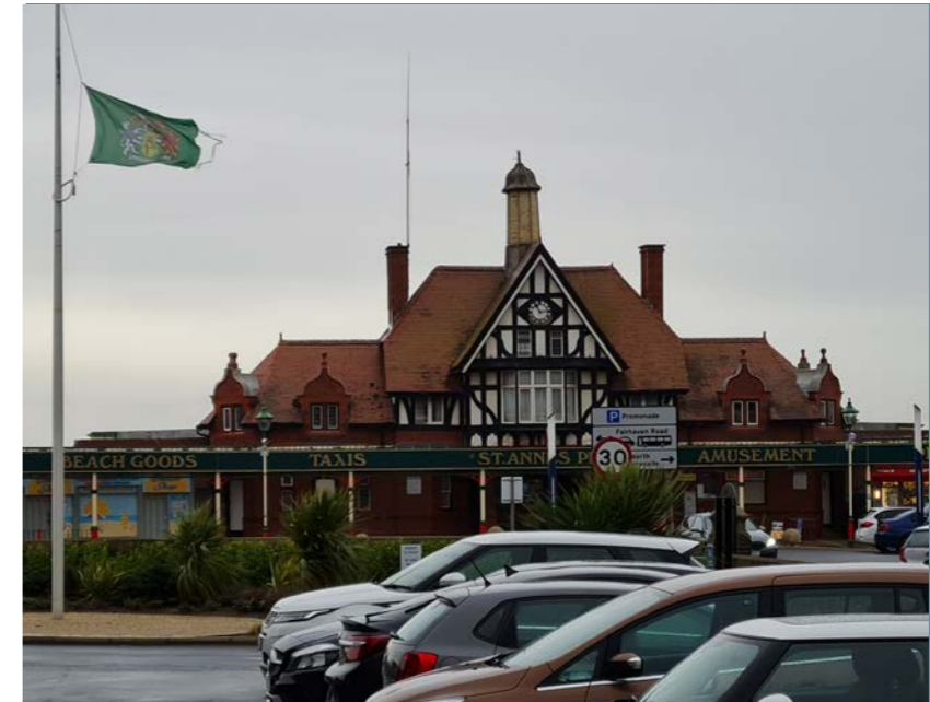
Heritage Assets (St Anne's Pier)
