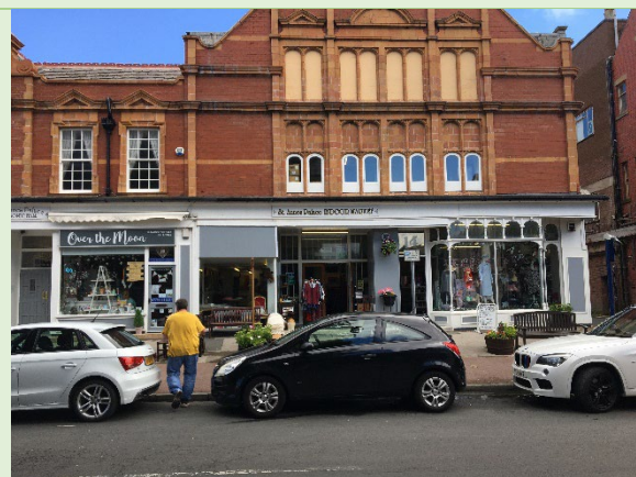
Figure 2: There are a number of high quality, attractive shopfronts throughout St Anne's which add to the town's overall character and appearance
