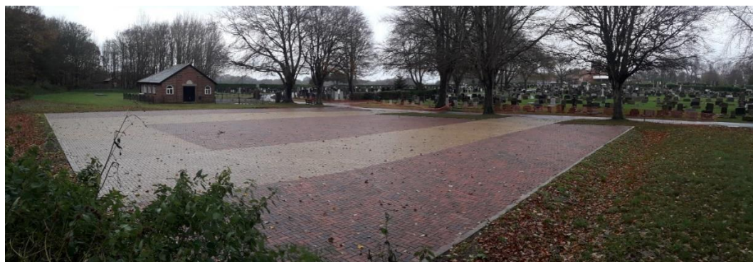
Figure 7: An example of permeable paving at Lytham Park Cemetery and Crematorium
