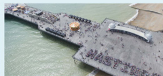
Hastings Pier - an example of how a pier can become a major public space
