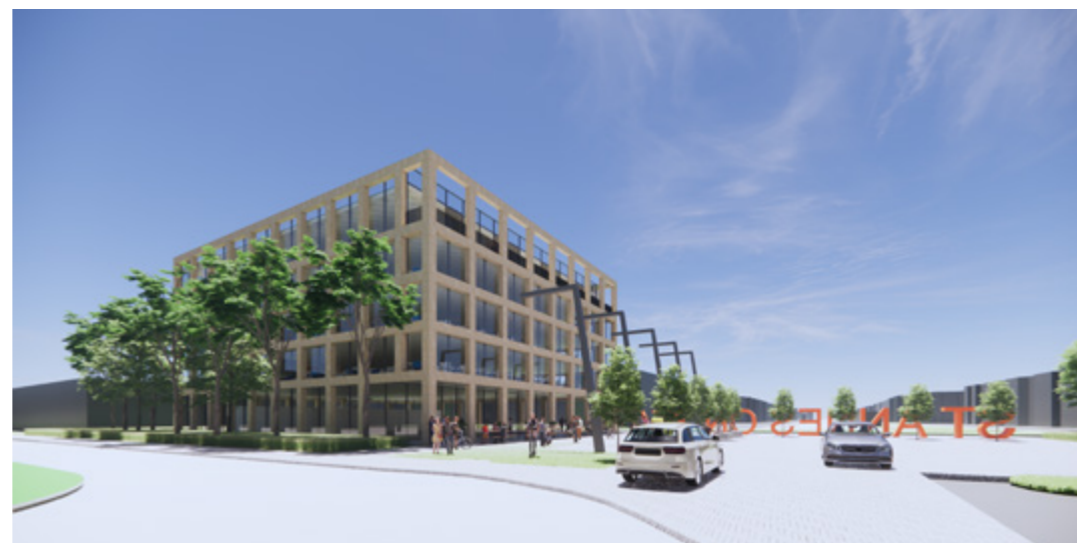
Figure 6.6: Station Gateway – view from St Andrew's Road North
