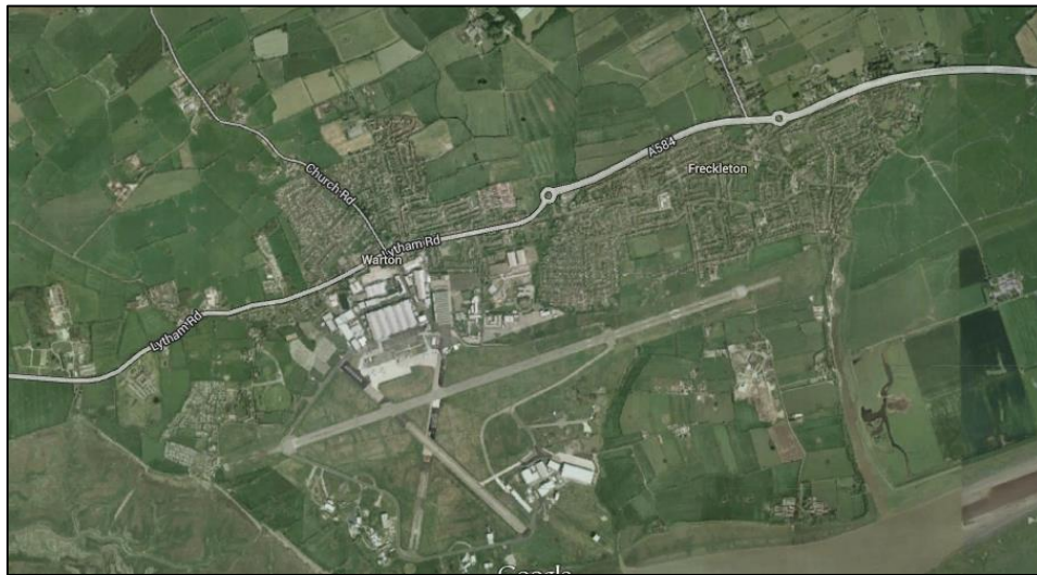
Figure 2.1 – Aerial of Warton and Freckleton
